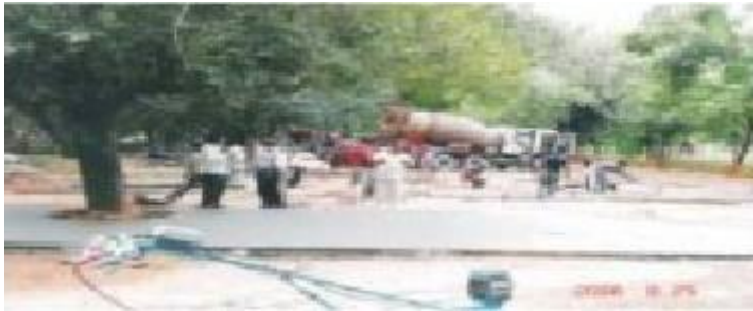
Figure-3: Laying of PFRC in parking over WBM surface
