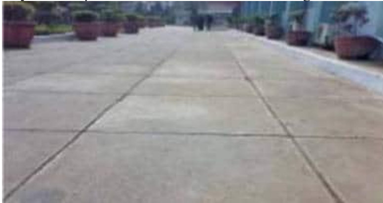
Figure-1: Pavement with steel fiber reinforced concrete
