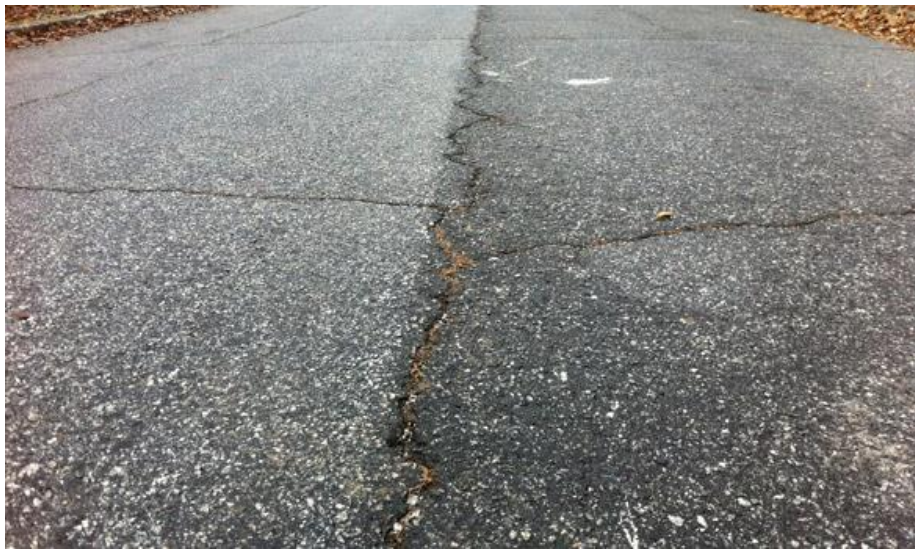
Figure 3.7 Longitudinal cracking
