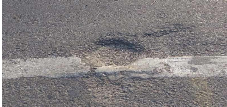
Figure 3.10 Potholes
