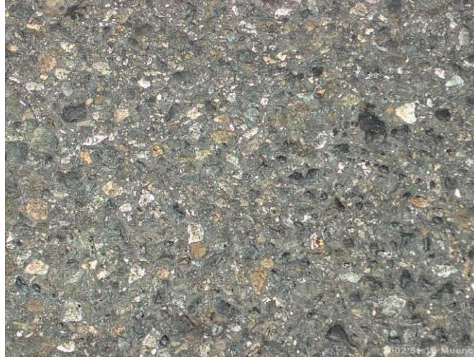
Figure 3.9 Polished aggregate
