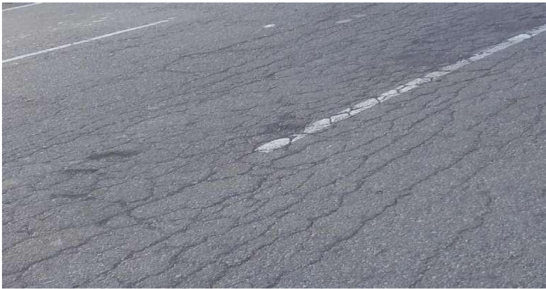
Figure 3.1 Alligator Cracks
