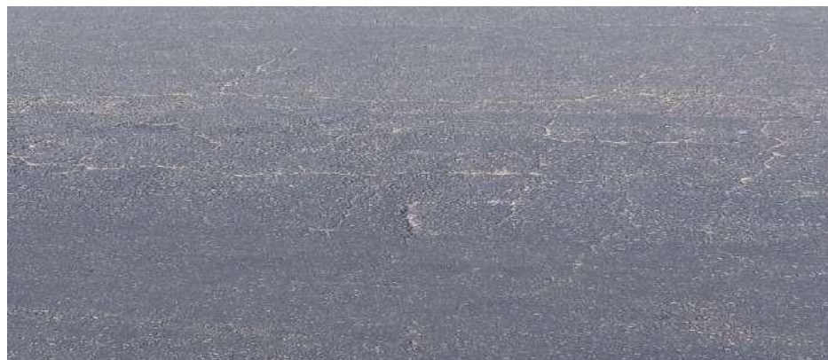
Figure 3.3 Block Cracking
