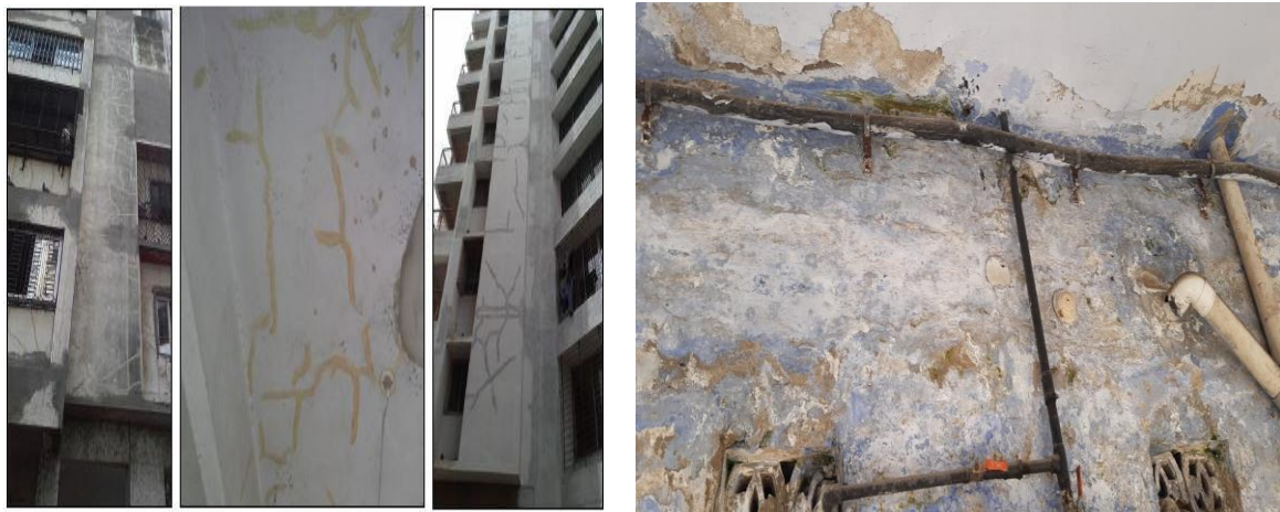
Fig. : Repair of cracks by Grouting method
