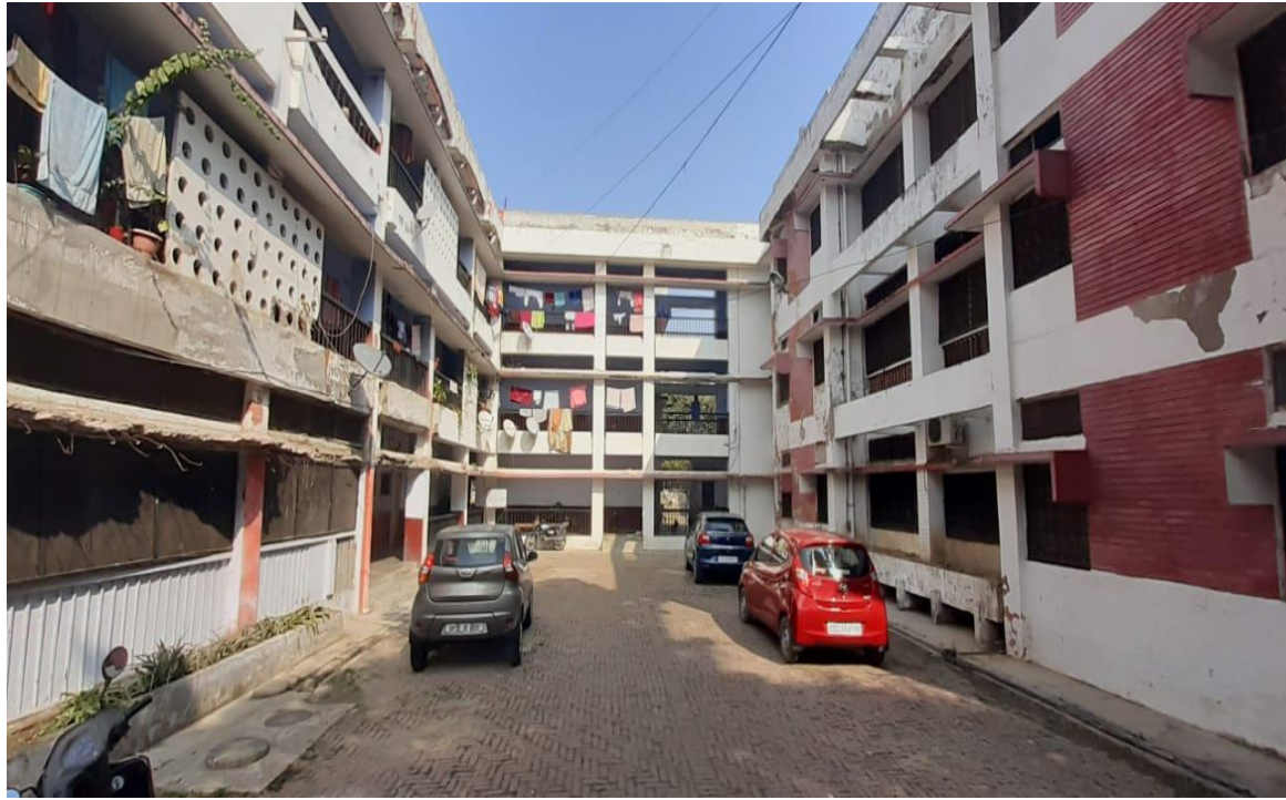
Plate 1. Front view of the building
