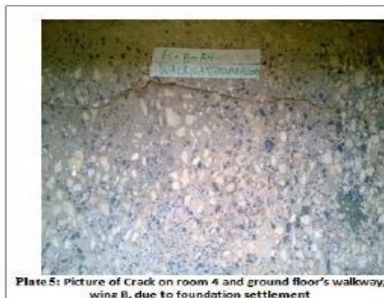
Plate 6: Picture of cracks on room 4, wing B, due to foundation settlement
