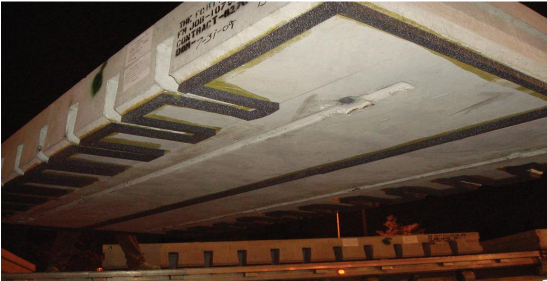
Figure 3.6. Proprietary grout distribution channels and gasket material on a Super-Slab JPrCP panel.
