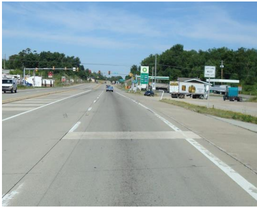
Figure 3.1. Concrete pavement with ramp Construction
