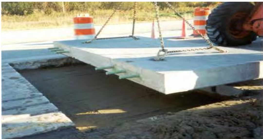
Fig 1.3 panel installation site view
