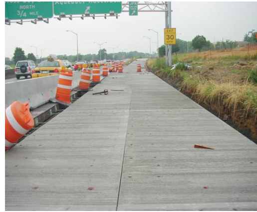
Figure 3.2. Wide precast widened concrete pavement
