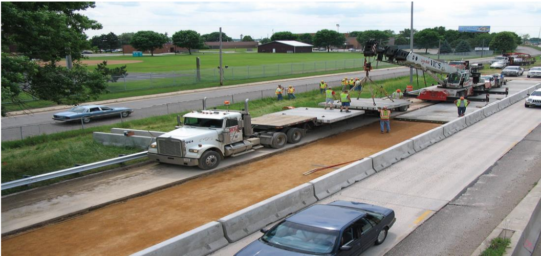
Figure 1.7. Example use of two lanes to perform repairs in a single lane
