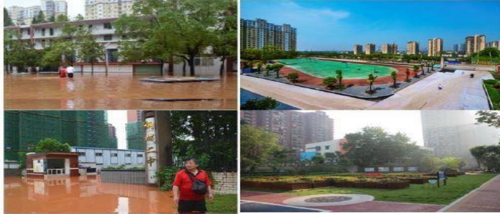
Figure 2.7 Before and after sponge construction of demonstration project – the Gangcheng No.2 Middle School in Qingshan district, Wuhan (Kang Dan, permissions from the Wuhan Urban and Rural Construction Bureau)
