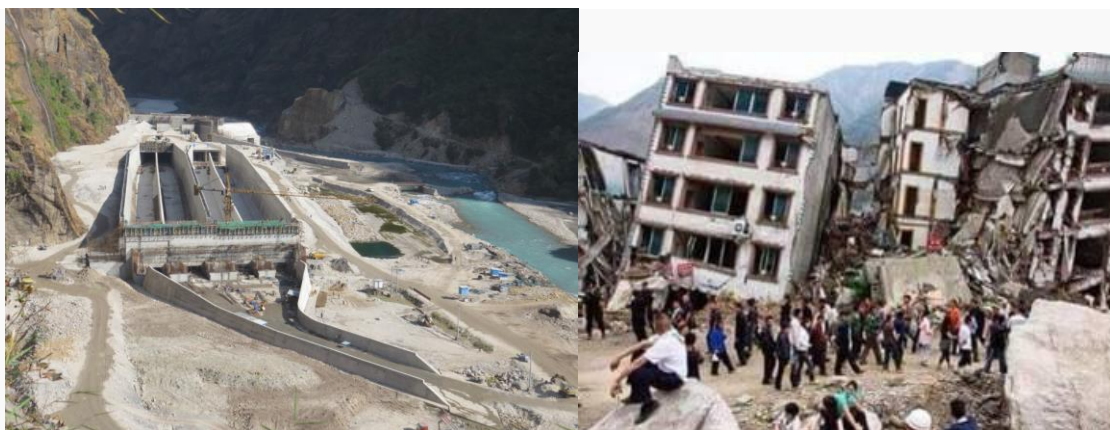
Upper Tamakoshi HEP under construction, it was damaged in the earthquake
