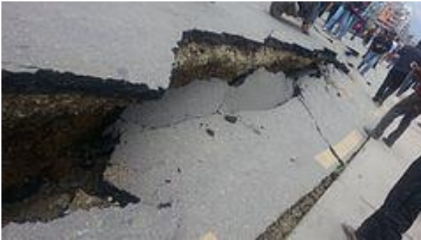
Road damage in Nepal
