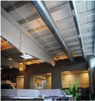
EXPOSED DUCTWORK AND SUSPENDED ACCOUSTIC PANELS
