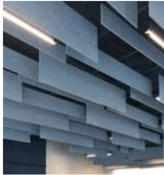
EXPOSED DUCTWORK AND SUSPENDED ACCOUSTIC PANELS
