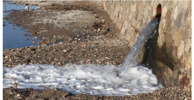
Figure 10.11 Sewer connection to the drain
