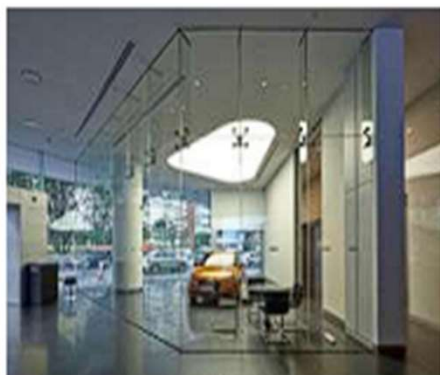
GLASSAND GYPSUM FALSE CEILING
