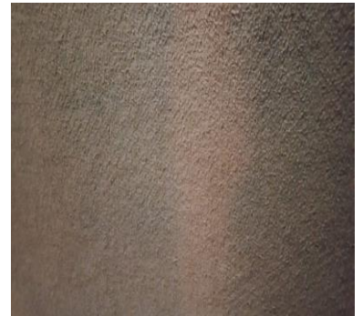
WALL FINISH IN AUDITORIUM
