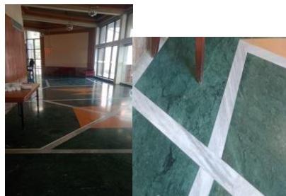
MARBLE FLOORING IN LOBBY
