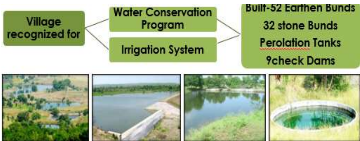
Figure 10 Earthen Structure, Percolation Tank, Check Dam & Open Well
