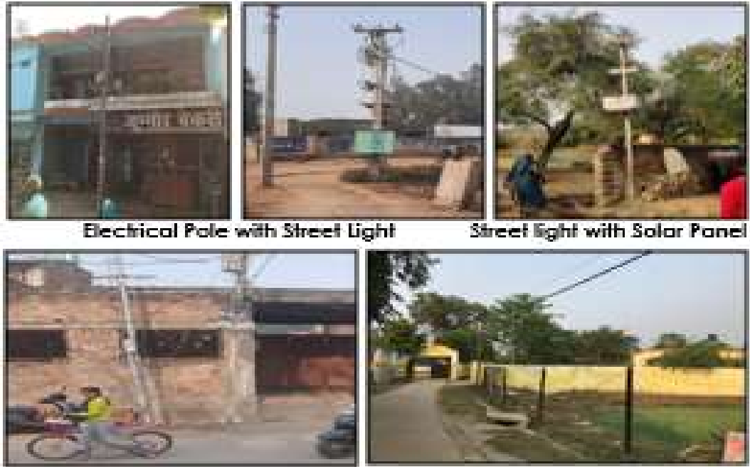
Figure 28 Electrical Poles in Juggaur Village
