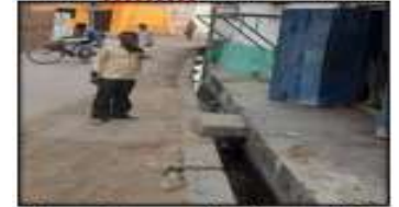
Open Pacca Drainage Line
