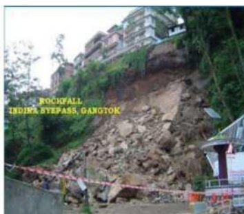
Indra Pass Road Landslide view
