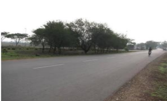
Fig. 3 Ramayanapuram Village Road (Corridor-3)
