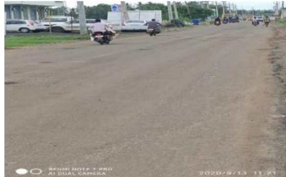
Fig. 2 Undi Bypass Road (Corridor-2)
