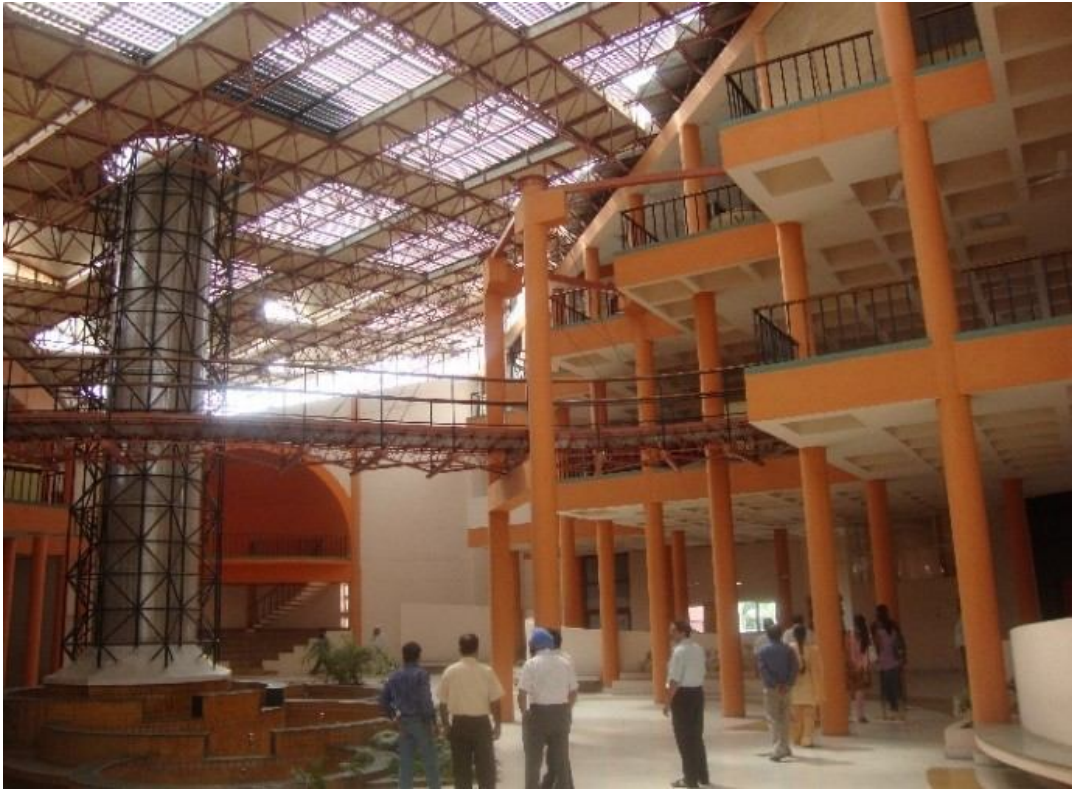
Figure 28. Atrium and Roof system
