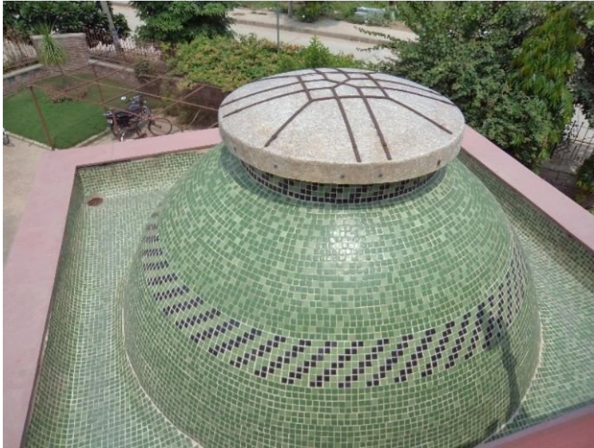
Figure 15. Ceramic Tile and Fiber material on the roof of the dome
