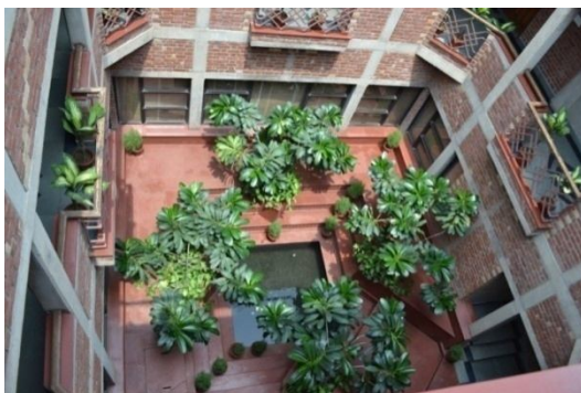
Figure 12. Sunken Courtyard at the Main entrance
