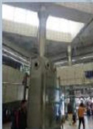
RCC AND STEEL COLUMNS TO SUPPORT THE HEAVY STRUCTURE
